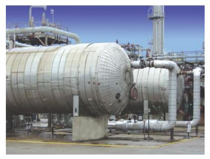
Storage and cleaning containers for alkylation units include fresh and discarded acids and water, acid analyzer settling tanks, and several sinks. Lye can neutralize free acids released in the reaction zone and neutralize alkyl sulfate in the net effluent. Washing breaks down the rest of the ester and removes corrosive agents and salts that may be produced from the alkali washing.
